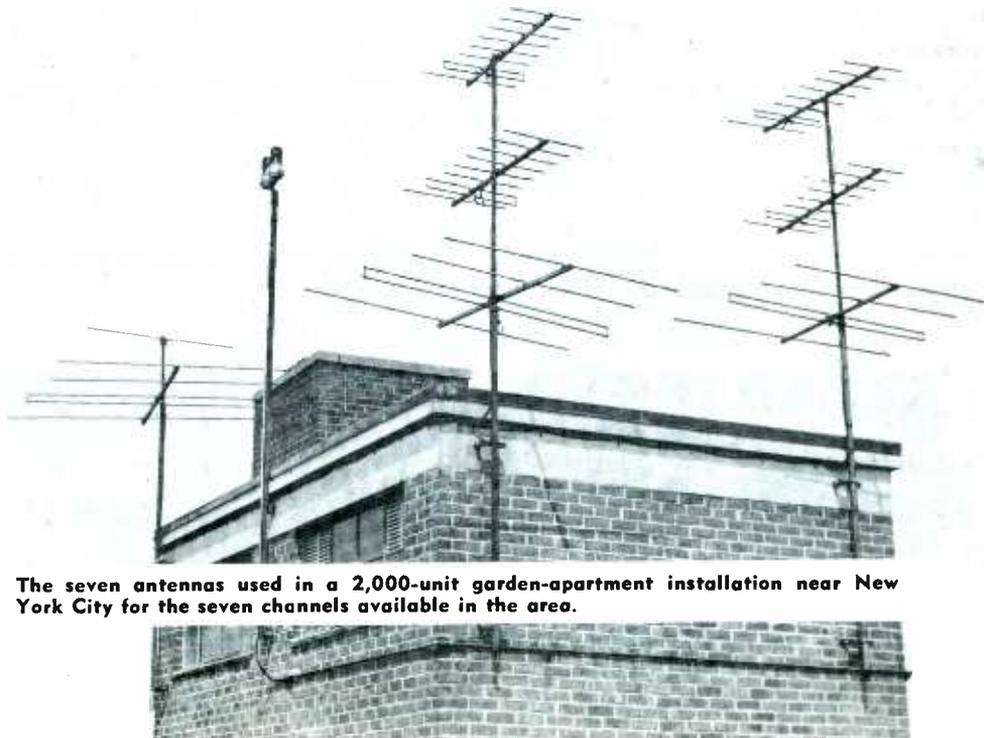
The seven antennas used in a 2,000-unit garden-apartment installation near New York City for the seven channels available in the area.
