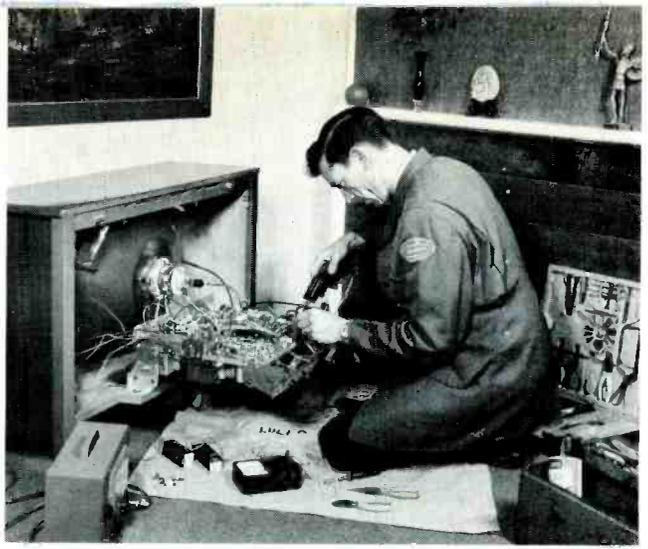
**Fig. 1** Because removing set from home increases the cost of contract servicing, as well as causing customer dissatisfaction, 97 percent of servicing performed by Hills is accomplished in the home by field technicians, as shown here. Average time in home per call is 38 minutes.
