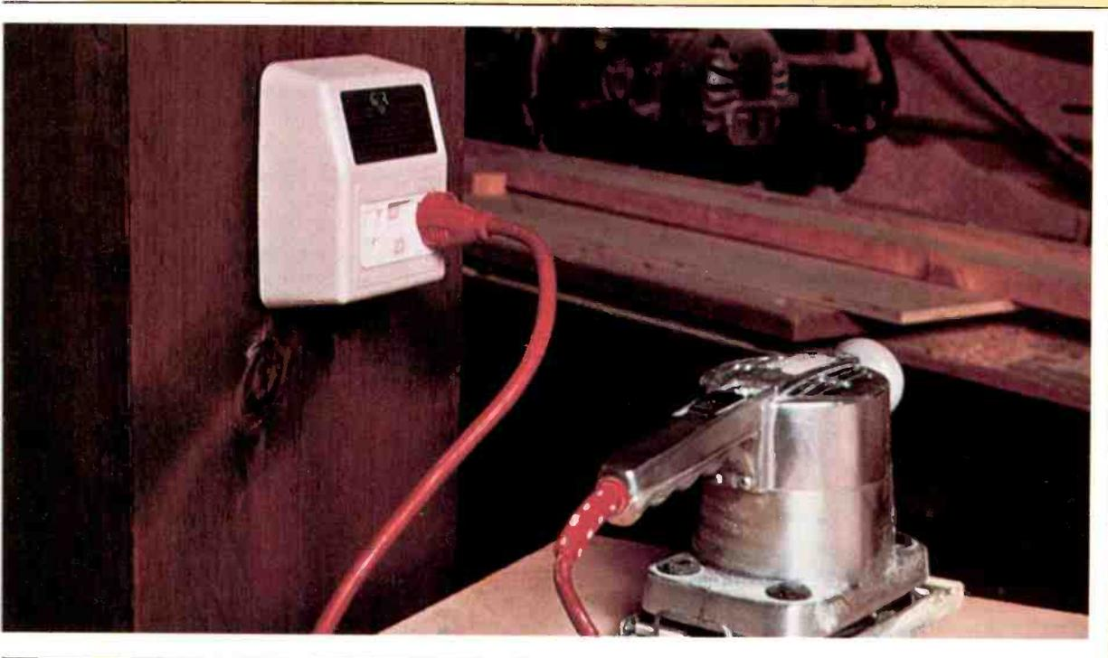
A plug-in GFCI gives portable current leakage protection.
