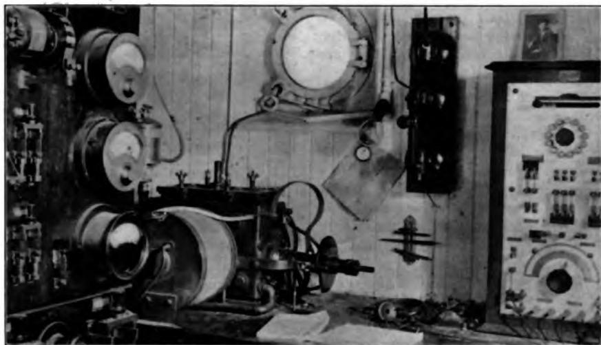
FEDERAL TRANSMITTER AND RECEIVER ON THE S. S. LANSING
