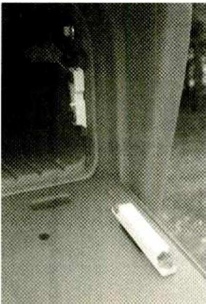
This closeup of the reed switch installation shows the liberal use of two-part epoxy to secure the switch and magnet in place.
