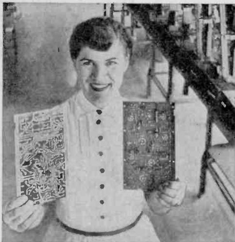
When all components have been mounted on printed circuit board, the underside is dipped in molten lead solder as in photo at right. This connects crimped ends of leads to copper pattern of printed circuit.
