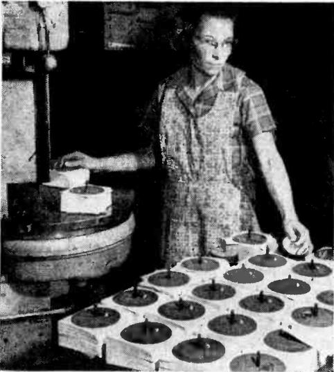
**8** Printing of labels, jackets, etc. undergoes careful editorial scrutiny. Copy must be grammatically and factually accurate. Color registration must be perfect. Labels are printed on large sheets and then cut to size on this machine.
