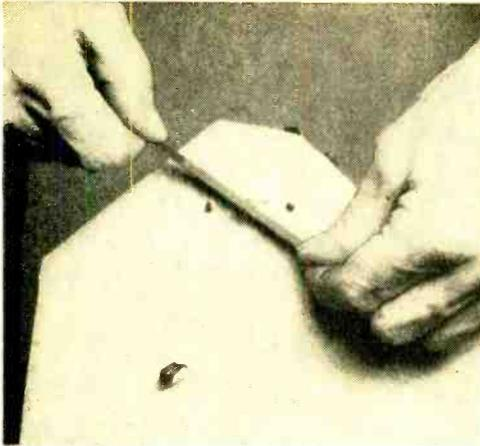
Fig. 3. File against the turn of the revolving shaft, using long, light strokes.
