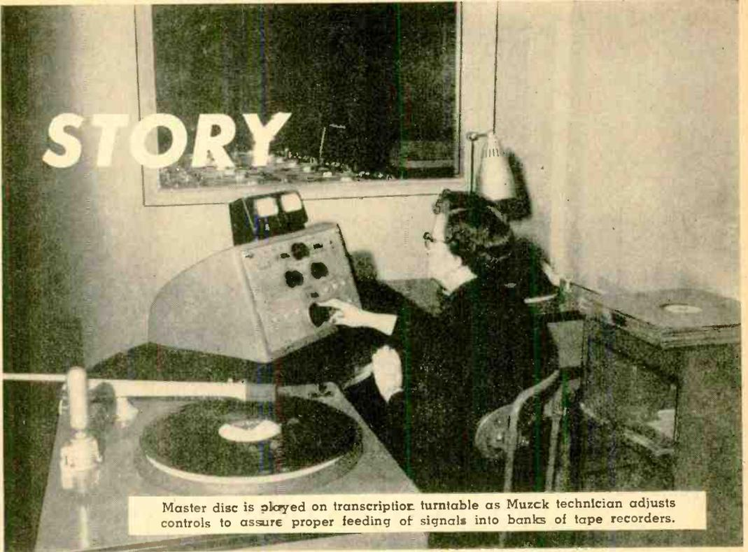
Master disc is played on transcriber turntable as Muzak technician adjusts controls to assure proper feeding of signals into banks of tape recorders.
