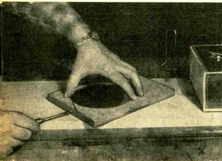
Cut a hole for the mirror with a jig saw. The diagonal cut in from the edge can be squeezed together with a screw to give clamping action in order to hold mirror in place. If mirror is loose in the holder, wrap layers of tape around rim until snug.
