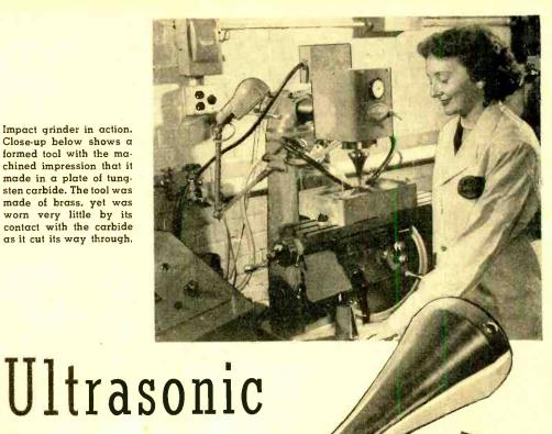
Flectronic tool machines hardest materials without contact
