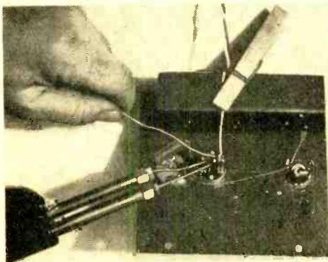
ing operation, you will appreciate this simple "kink." When you get your wire in the desired position, put some tension on it and clamp it in place with a spring-type clothespin. Use one for each wire if you are making a multiple connection.
