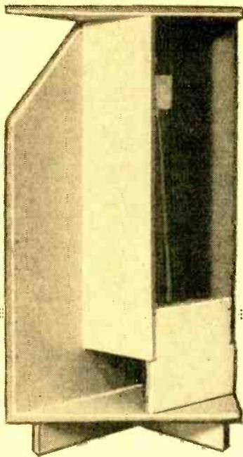
Rear view of enclosure shows placement of the various Celotex sections.
