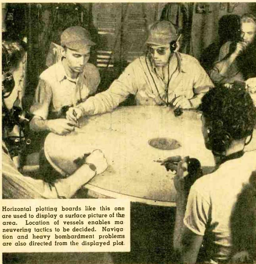
Horizontal plotting boards like this one are used to display a surface picture of the area. Location of vessels enables maneuvering tactics to be decided. Navigation and heavy bombardment problems are also directed from the displayed plot.
