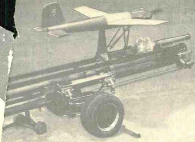
of small drone air-planes may be done in a number of ways. Above, a catapult is being used to provide Navy target drone with JATO assist.
