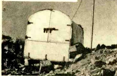
transmitting it on a "clear channel." The Translator includes a v.h.f. antenna, v.h.f. tuner, v.h.f. to u.h.f. converter, u.h.f. amplifiers, u.h.f. antenna, and an automatic code identifier. A single cabinet houses all this gear. Antenna combinations handle various powers and special radiation patterns. Because the Translator's output is confined to the less-congested upper end of the u.h.f. band, the FCC has granted approval for the system.
