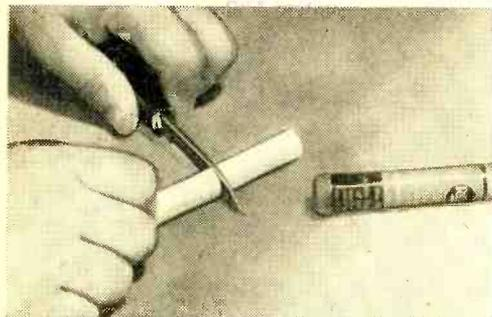
**Operating power** for the simple receiver is supplied by an 11.2-volt battery, made up by cutting an eight-cell section from an RCA Type VSO87 "separable cell" battery. You can easily cut out the desired section with an ordinary pocket knife.
