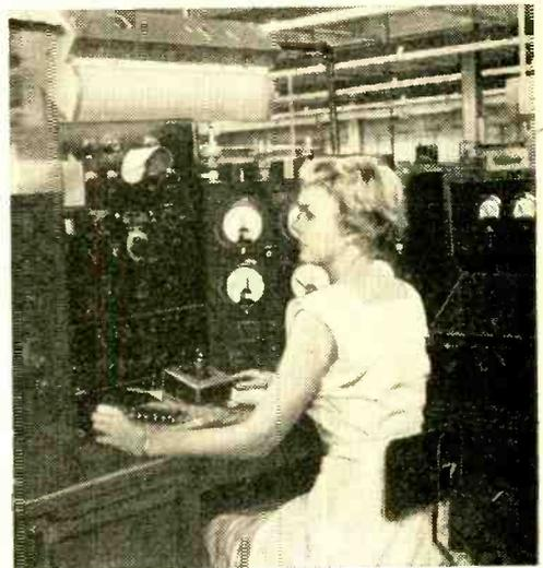
**Quality control programs** supplement regular production testing to make sure that all tubes sold under brand name meet specifications. Scientific sampling techniques validate spot testing.
