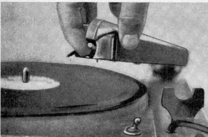
Like the cutting tool of a lathe, the stylus cuts the groove into the blank. It should be sharp, as shown (top). With no signal on cutter, grooves should be smooth and concentric as in photo A (center); in B, you will see "wiggles" cut by stylus as sound is applied to mike. The blank must be moving on turntable before stylus is placed on it. Start first cut  $3/16$ " from edge of blank or previous recording, as shown in bottom photo.
