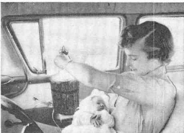
**Electronic bottle** cooler-warmer, with no moving parts, plugs into car's cigarette lighter. Fifty thermoelectric junctions cool or heat the bottle instantaneously. The current that produces cold can be reversed to produce heat for cooking. This experimental Westinghouse device has vertical aluminum fins for air cooling or dissipation of removed heat.
