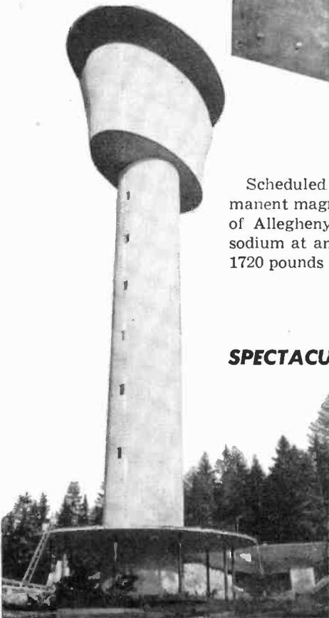
A new ultra-modern TV tower has recently been built near Heidelberg in West Germany. The 124-foot structure has an observation tower for visitors and a tank for storing drinking water. An antenna placed atop the tower will make the total height of the installation 258 feet. (Wide World photo)
