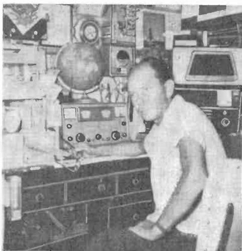
**Anson Boice, WPE1BD,** works with a Hammarlund HQ-100 and a Grundig receiver. His current equipment also includes a Webcor tape recorder and a POP'tronics antenna tuner.
