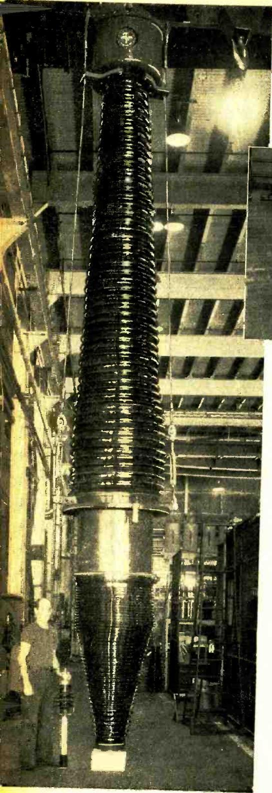
**Combination** turbine and generator units (below), part of the Consolidated Edison Company's Astoria, N. Y., station, can generate up to 360,000 kilowatts. Huge 650-kilovolt bushing (left) is destined for service in the General Electric Company's experimental extra-high-voltage line between Lee and Pittsfield, Mass.; weighing 10,000 pounds, the 28-foot unit dwarfs workman holding a 23-kv. bushing.
