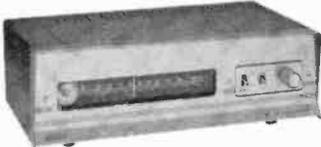
**ST-25 FM TUNER:** Sensitivity: 1.5 microvolts for 20 DB quieting. Harmonic Distortion: less than 1%. Includes: Dual Limiters, AFC and AFC Deaf, "Eye" type tuning indicator, Multiplex Jack. Black and gold case or walnut enclosure at slight extra cost.
