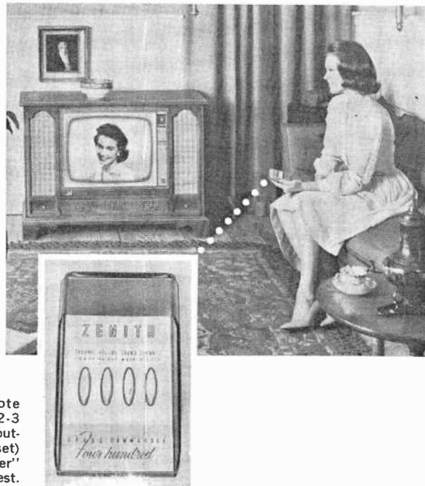
Fig. 1. Transistorized remote control is now simple as 1-2-3 on many new TV sets. Press a button on the "transmitter" (inset) and a transistorized "receiver" in the TV set does all the rest.
