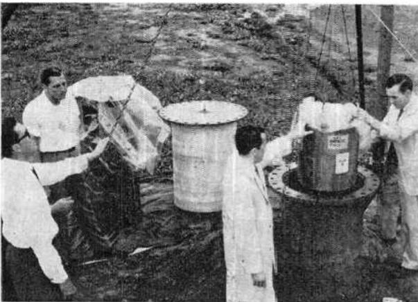
Generator for power station is lowered into half-buried cylinder during tests at Baltimore, Md., plant of the Martin Company. Unmanned station will operate without maintenance or refueling for two years once it is completely assembled and fully sealed.
