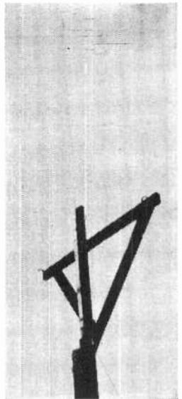
Front and side views of completed antenna clearly illustrate the simple construction. After mounting mast, complete the job by adding four 10' 6" radials. These are cut from #12-#16 copper wire, and each is terminated in an insulator.
