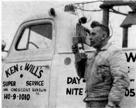
Within the past year, a new type of CB transceiver has put in an appearance—the 1-watt hand-held portable unit. This tow truck operator is using a new Knight-Kit (Allied Radio) to contact his base.
