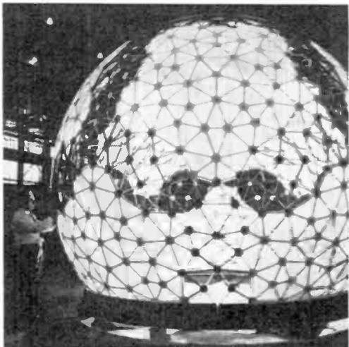
**BLAST DOME**—Radomes designed to protect radar antennas from shock and blast as well as from the weather are being produced by Goodyear. The structures get their strength from unusual geometric configuration; skin is fiberglass.
