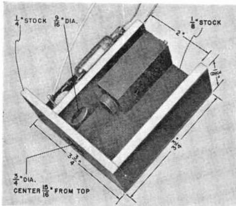
Light-source barrel is made from a block of wood. Size of lens opening can be varied to accommodate your lens. Use a cardboard tube as an extension.
