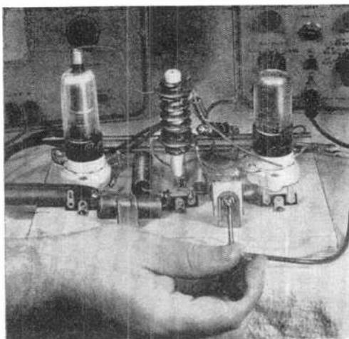
Fig. 1. All parts of this "classic" breadboard are readily accessible. Tests and adjustments are made conveniently from top of "chassis."
