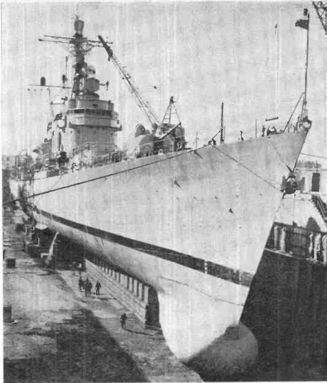
**GIANT RUBBER NOSE**—Big as a bungalow, and weighing nine tons, rubber nose attached to keel of U.S. Navy Destroyer "Willis A. Lee" is actually a giant sonar dome which protects sensitive sonar equipment housed below ship's water line. Made by B. F. Goodrich Aerospace and Defense Products, the dome has inch-thick rubber walls with acoustical properties similar to those of sea water, permitting sound to pass through with minimum distortion.
