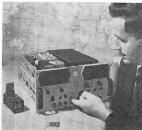
**LOST AT SEA?**—Containing transistorized microcircuits fabricated by ITT Federal Laboratories, miniature "Omega" receiver enables a ship to determine its location within half a mile at a distance of 5000 miles. These receivers are being built for use on U. S. Navy vessels around the world.
