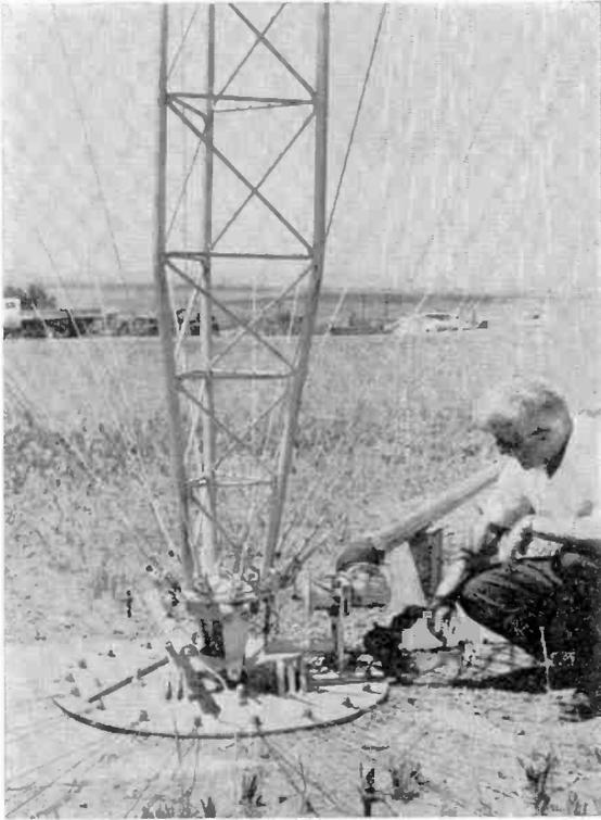
**WWV RELOCATES**—Construction is nearly completed on the new WWV transmitter building and control center at Fort Collins, Colo., from which the NBS standards broadcast station is scheduled to transmit beginning in December. Photo shows standby antenna fed by  $3\frac{1}{8}$ " coax line.
