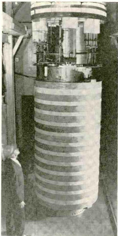
**GIANT MAGNET**—What is believed to be the world's largest superconducting magnet, shown on display at Avco Everett Research Laboratory, produces 40,000 gauss over a 5' x 12" field region. Weighing 15,675 pounds, the giant magnet stands 10' high, and stores 5,000,000 joules of energy. Designed for use in a magnetohydrodynamic (MHD) power generator, the saddle-shaped magnet was made possible by a recently developed (by Avco) "stabilized" composite superconductor.
