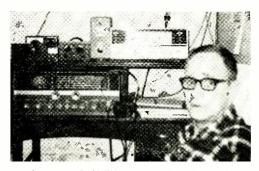
Leo Stowell, WPE9HTU, has a well-equipped listening post in Chicago, III. In addition to a Hallicrafters S-108 receiver, there is an antenna tuner, an Smeter, a nuvistor converter, a 6-meter converter, and another Hallicrafters receiver, an S-120.
