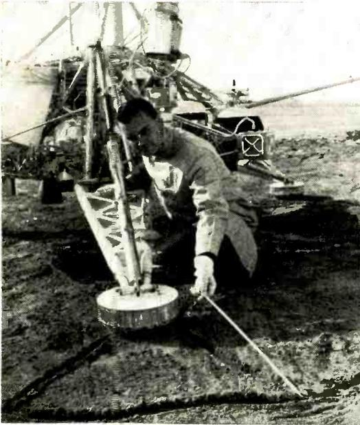
**SOFT LANDING VERIFIED**—With data taken by electronic strain gauges made by Baldwin-Lima-Hamilton Corp., Surveyor 1's soft landing on the moon was verified and radioed back to earth. The strain gauges also provided important data on the bearing strength of the lunar surface.
