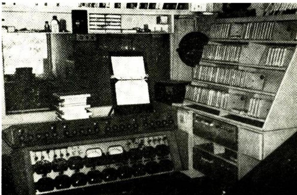
Operating at 1160 kHz on the standard broadcast band, and 6000 kHz on the international broadcast (short-wave) band, Radio Americas routes all program material through control console shown at lower left.
