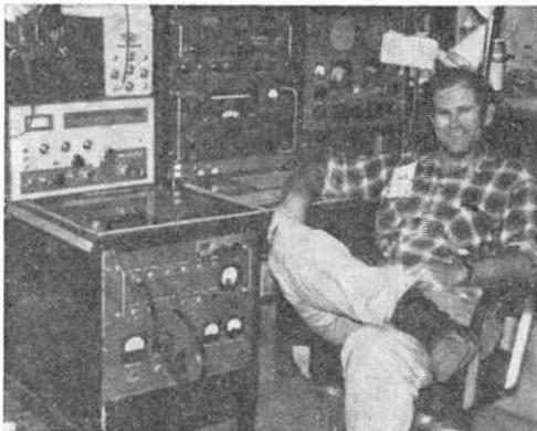
Walter H. Trefzt, KL7GGU, Anchorage, Alaska, has a well-outfitted station with, on the table, left to right, a Heathkit Apache/SB-10 transmitter and Collins 51-J3, Hammarlund SP-600-JX, and Hallicrafters S-36 receivers. Antennas—a 10/15/20-meter beam and 80- and 40-meter dipoles. He didn't identify the unit at lower left—possibly an antenna tuner?
