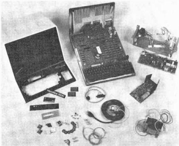
*Hazeltine's Model 1500 computer terminal comes in semikit form as shown here and is easily assembled.*
