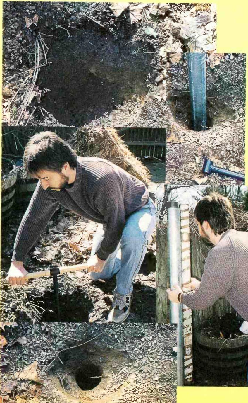
prevent the post from turning. Four additional metal pieces are attached to the clamps to act as guides for the Qik-Base's angle-iron "roots." Then the roots are pounded into the earth, the hole is filled, the sod is replaced, and you've got one sturdily mounted pole!
