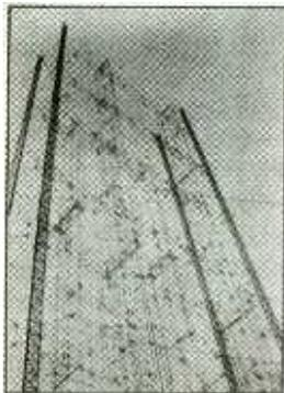
Curtain antenna with eight parallel-fed dipoles, 20M for special event.
