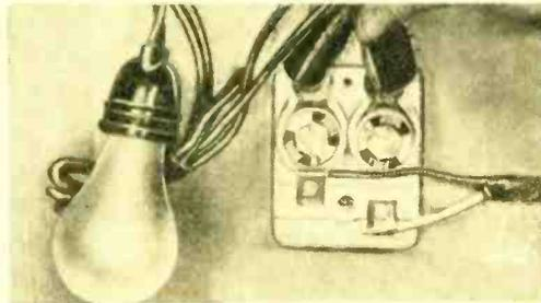
Occasionally it is difficult to see whether a fuse has blown. To "cross-check" fuses, remove one and tap the test lamp from the input to appliance side of fuse (above, left). If the light glows, the fuse removed is burnt out.
