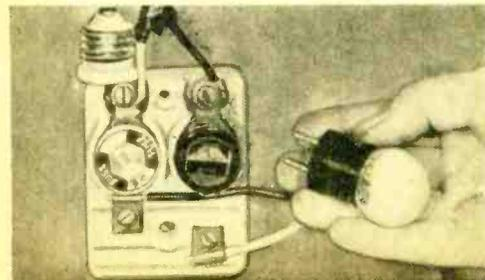
A low-amperage ground often eats up current without notice. To check for such a ground, turn off all electrical gadgets in the house, and insert the connector plus bulb (left). If bulb glows, the ground indicated should be located quickly to prevent a fire hazard.
