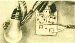
Occasionally it is difficult to see whether a fuse has blown. To "cross-check" fuses, remove one and tap the test lamp from the input to appliance side of fuse (above, left). If the light glows, the fuse removed is burnt out.
