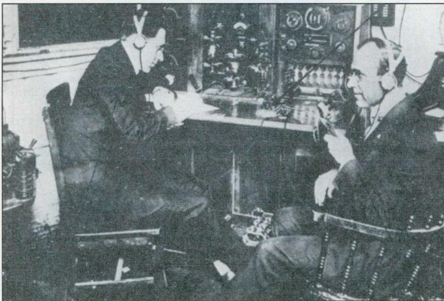
*This early photo of XWA shows the transmitter to the left, the receiver at the right, and a telegraph key in the desktop's center. The operator seated to the right is holding a microphone.*
