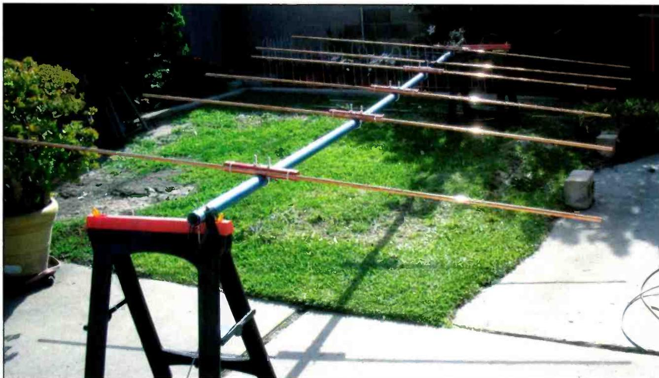
*Photo D. The beam is initially assembled on the ground, to assess mechanical integrity and to get the elements level.*
