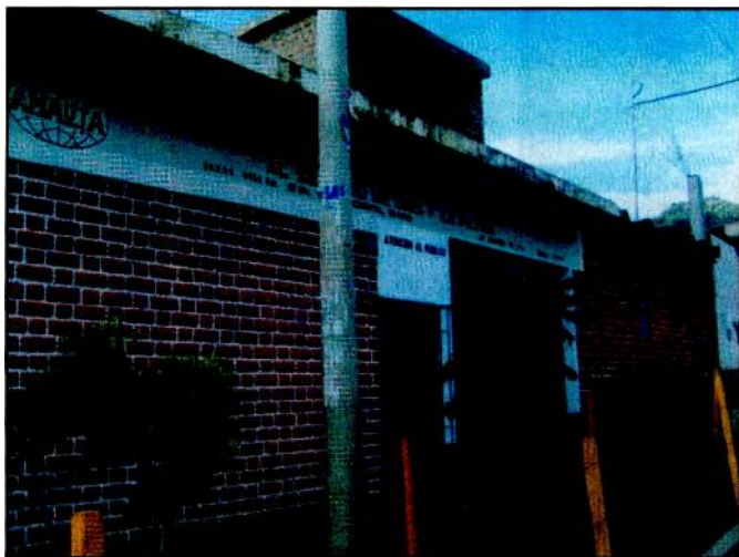
Radio Cultural Amuata broadcasts from this building in Huanta, Peru. It's on 4955. (Thanks Rich D'Angelo, PA)
