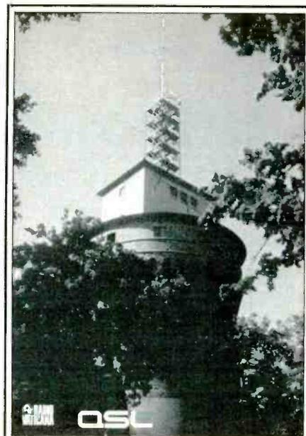
This antenna installation on the Tower of Leo XIII provides the radio link between studios and the Santa Maria di Galeria site.
