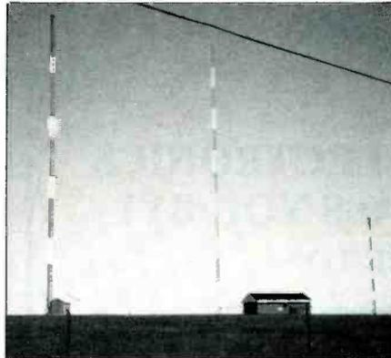
*The transmitter building and antenna system of CJLS, Yarmouth, Nova Scotia, Canada. This station operates on 1340 kHz with 5 kW. The transmitter and antennas are located at Shebouge Harbor near Yarmouth. (Photo by K. Kneitel)*
