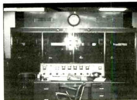
Here is a shot of the 26-year-old WBAL 50-kW transmitter which has just been replaced with a new Continental. This is an RCA 50H Ampliphase with a solid-state exciter. The consol at the front of the picture is left over from the original 50-kW Westinghouse installed when the building was new in 1941. The transmitter still runs fine but the clock has died!
