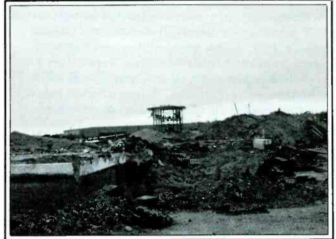
**AFTER:** It took only one day to convert the transmitter building into this mound of rubble. In the background you can see a structure that served as a distribution point for feed lines to go between the transmitters and various antennas.
