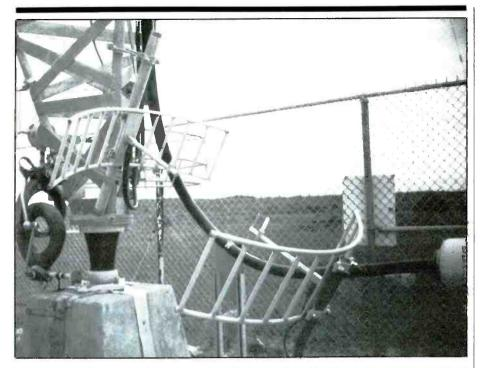
Fig. 6- Base of antenna. Note system of reflector backed dipoles used to couple studio to transmitter link system to antenna on the tower. Interlocked rings on left is the air core transformer for the tower obstruction lights. Ball tipped rods are the lightning protection spark gap. The dark colored cone shape item is a ceramic insulator, it is the sole support for several tons of tower.
