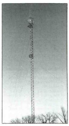
A construction company rents space on this tower for their 43.12 MHz antenna. The office is linked to the tower on 75.72 MHz.
