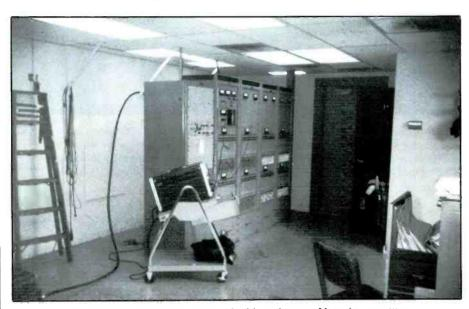
Fig. 8- Interior of TUK's transmitter building showing Nautel transmitters.
