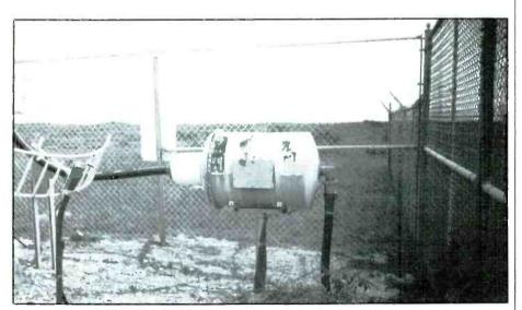
Fig. 7- Isocoupler used to couple FM antenna on top of TUK antenna to transmitter. It isolates tower from ground and FM transmitter, and prevents interreaction of FM signals and TUK's signals.
