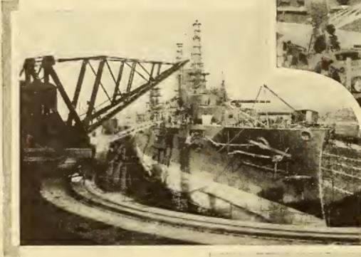
Fifty Ton Cranes Travel around the Ship on Rails
