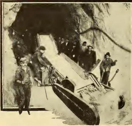
A Mucking Machine at Work in The Tunnels—Far Ahead of Hand Labor for Rapidly Removing Excavated Material from the Working Face
