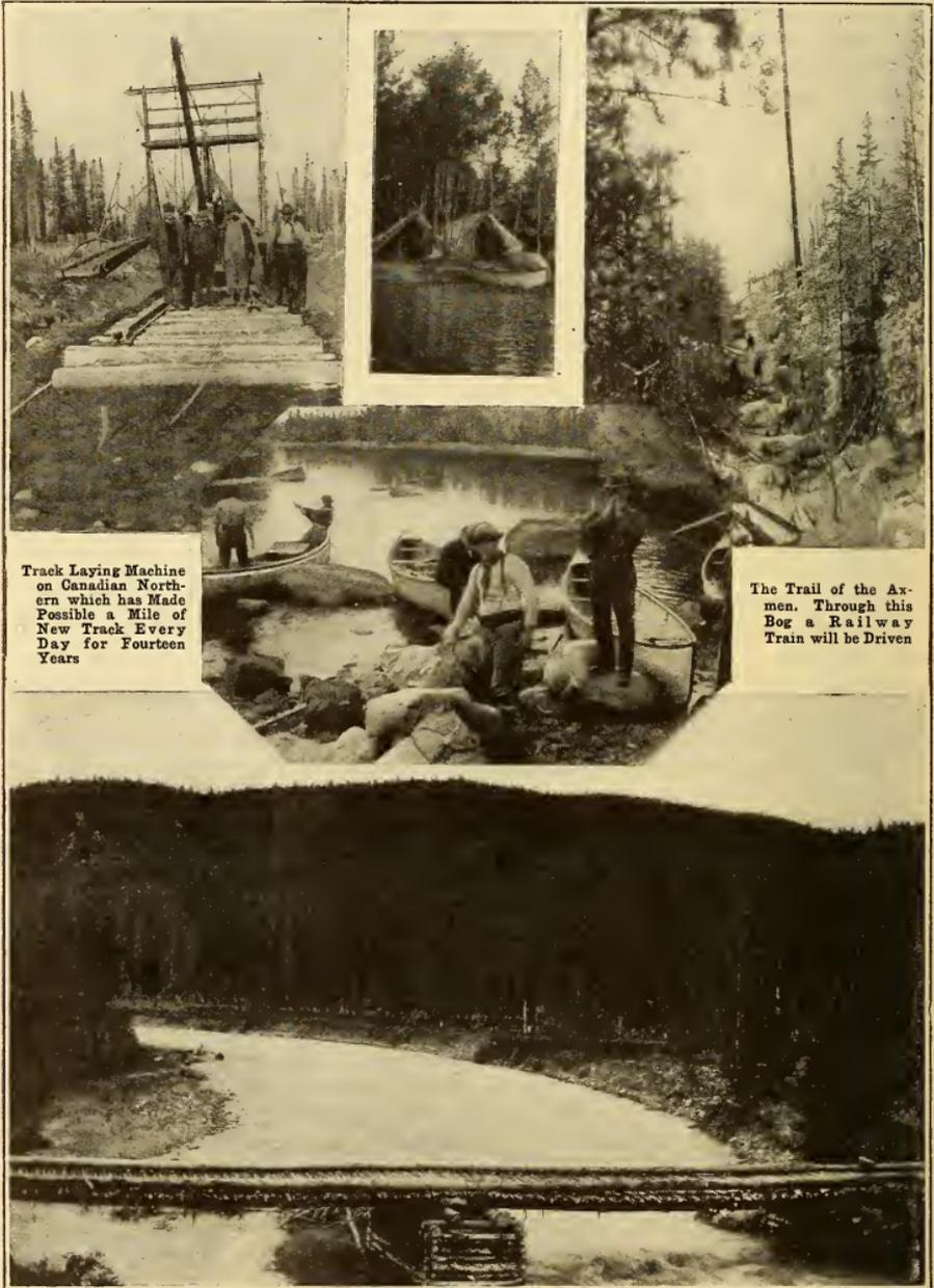
Track Laying Machine on Canadian Northern which has Made Possible a Mile of New Track Every Day for Fourteen Years
