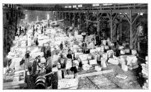
ELECTRICALLY DRIVEN BARREL SAWS AND FLUTING MACHINES GETTING OUT MARBLE FOR THE DENVER FEDERAL BUILDING
