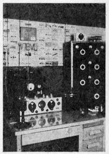
W7BVL, Dr. Dull's station in Seattle, Wash. The nine-tube superhet receiver and the 200 watt transmitter, as well as most of the other equipment shown, is home made.
