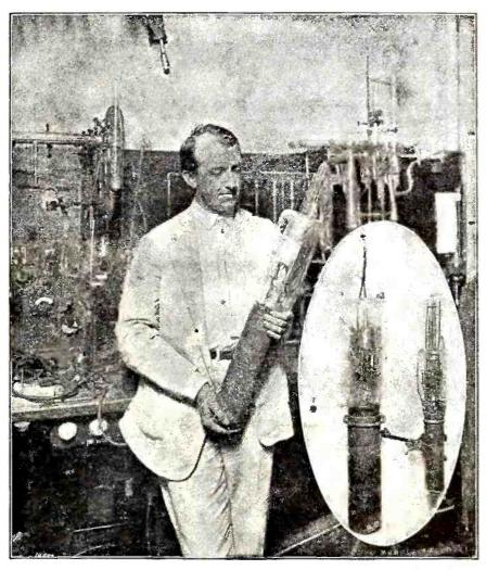
W. G. Houskeeper, the Western Electric engineer whose epoch making invention led to the production of the world's largest vacuum tube, and the tube itself. Insert shows in graphic fashion just how the new monster tube compares with the little "peanut" tube used in the average radio receiving set and the 10,000 watt tube which only recently was considered the last step in this department of science.
