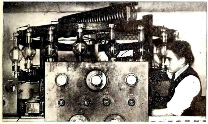
Giant transmitter at Station WJAZ, Chicago, showing the arrangement of big tubes in a circle. The studio of this station is enclosed in plate glass. (U&U Foto).
