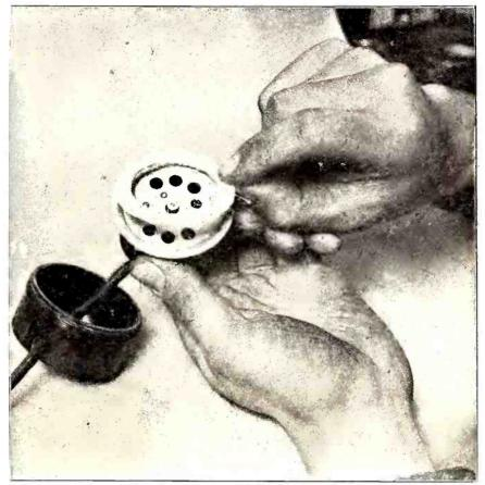
If there is a rattle in the phone when i, is used as a loud speaker, the trouble may be eliminated by placing a cardboard disc over the diaphragm as shown in the photograph. The cap of the receiver should then be screwed on until the quality of the tone is best. (Kadel & Herbert.)
