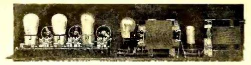
Fig. 2. A picture of the wiring arrangement of the Browning-Drake set. By bringing the terminals from the amplifier to the under side of the base panel, most of the wiring is kept out of sight.
