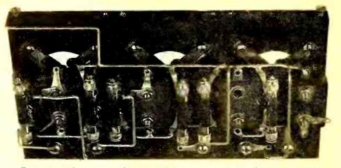
Figure 3. A bottom view of the amplifier, giving a good idea of how resistances and condensers are mounted.
