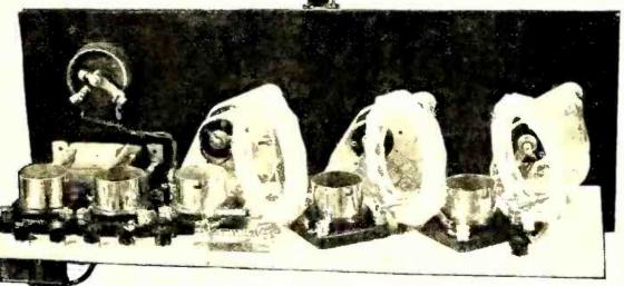
In the set above is shown the proper arrangement of coils to prevent inductive coupling. Engineers have made a study of the effect of the magnetic fields of adjacent coils upon each other, and efforts have been made to so place the coils in the receiver that the effect is reduced to a minimum. Radio experience also has shown that better results are obtained in reception if the aerial is pointing toward or away from the sending station sought. This is especially true of the loop aerial.
