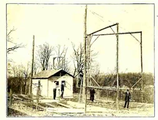
Figure 1. The photo, made by the Bureau of Standards, shows a double-coil transmitting device used for sending out radio signals whereby an airplane or ship may be guided along a straight course, thus taking the place of less reliable methods.
