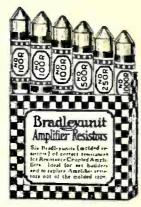
sistor is called, are molded in place. The Bradley unit does not rely upon hermetic sealing to avoid de-terioration. The silver plated contacts are pro-vided with holes for soldering, or they may be used in the standard mounting clip.
