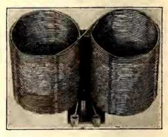
NOTHER product has been added to the Benjamin line with the announcement of the "Lekeless" r. f. transformer, made in binocular form, with self-supporting wire turns.
