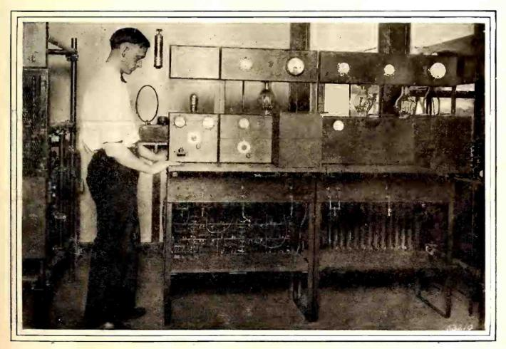
Fig. 3. KDKA controls its vast antenna output by means of the small crystal described by Mr. Winters in this article. The picture shows the crystal oscillator with a 5 watt tube in the panel in front of the operator
